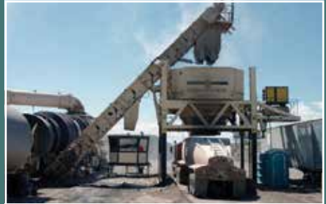
Lime in Asphalt
