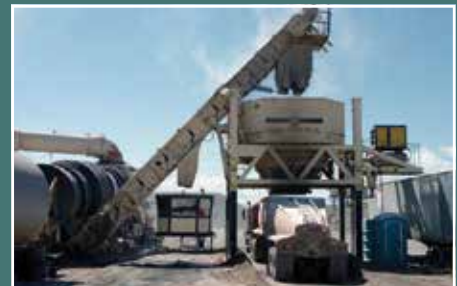
Lime in Asphalt
