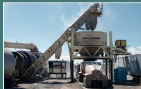
Lime in Asphalt
