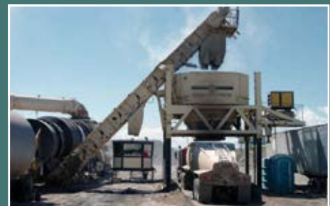
Lime in Asphalt
