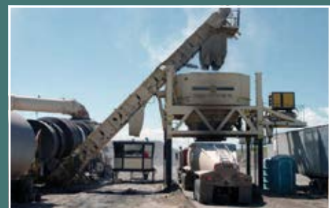
Lime in Asphalt
