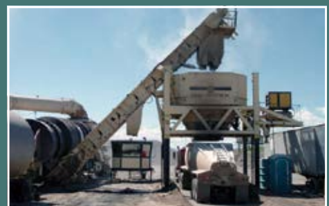
Lime in Asphalt
